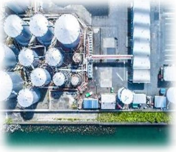
Petrochemical and Refinery
